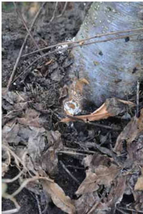
Figure 12. Mushroom root rot caused by Armillaria spp. in peaches shown with a cut in the bark near the soil line. Notice white hyphae just under the bark before cutting into the wood.
