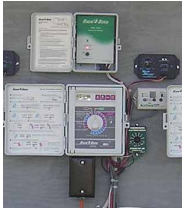
Figure 2. Four brands of soil moisture sensor controllers with an electronic time clock.
