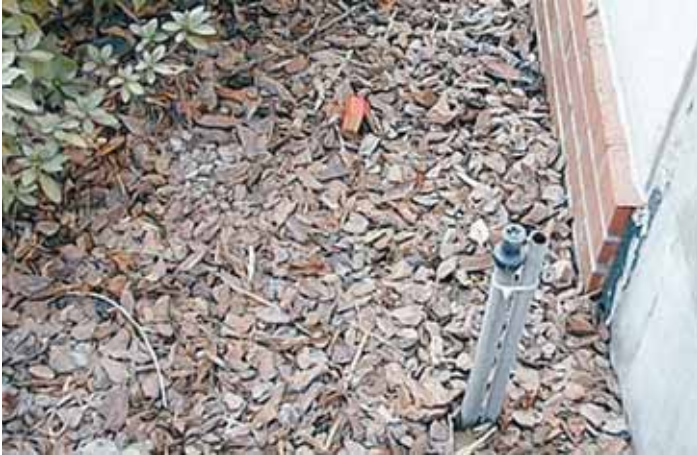
Figure 2. Mulch that is too thick and obscures an inspection space will result in what is termed a “conductive condition” in the pest control industry. Some termite contracts may become void with the presence of conducive conditions around a home. The irrigation head depicted here is in violation of the current building code. The Florida building code requires that irrigation be installed 1 foot or more away from a building sidewall. Irrigation heads that “water walls” is also considered a conducive condition.
