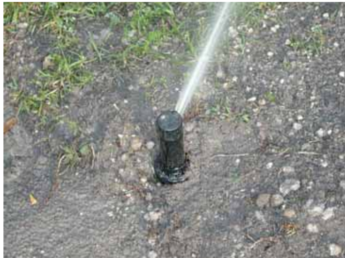
Figure 2. Gear-driven rotor irrigation head.
