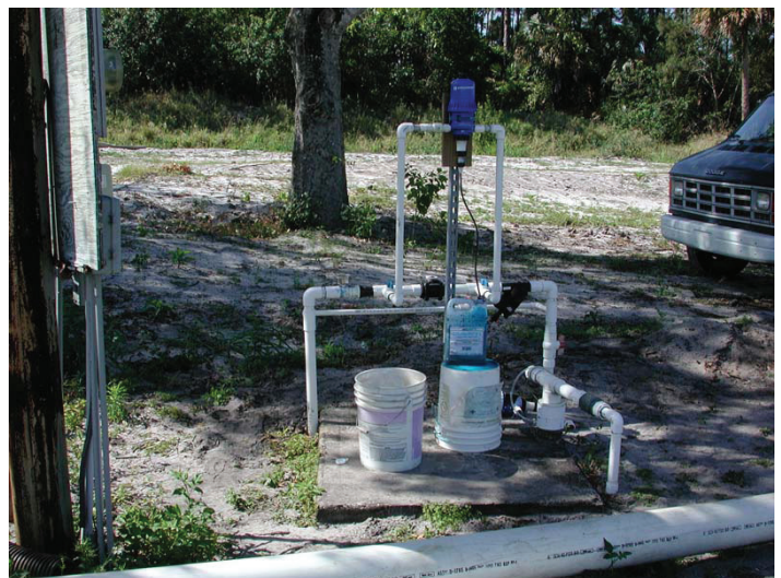
Figure 5. Injection made possible with a Dosatron. Credits: Eric Simonne.
