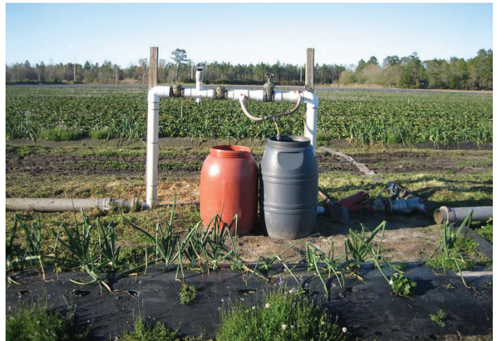
Figure 4. Back-flow prevention made of two ball valves and a vacuum breaker are placed upstream of the Venturi injector. Credits: Eric Simonne.
