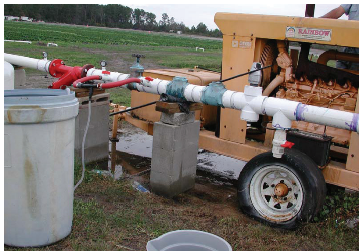
Figure 2. Diesel engines mounted on a trailer offer the greatest flexibility of use.
