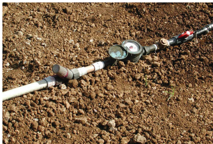
Figure 8. Water meters installed near the field.
