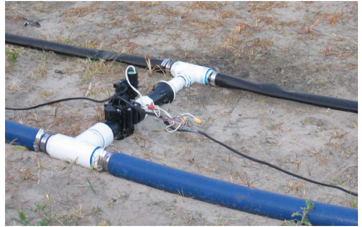
Figure 11. Solenoid valves connected to a timer allow sequential irrigation of different zones. Credits: Eric Simonne.
