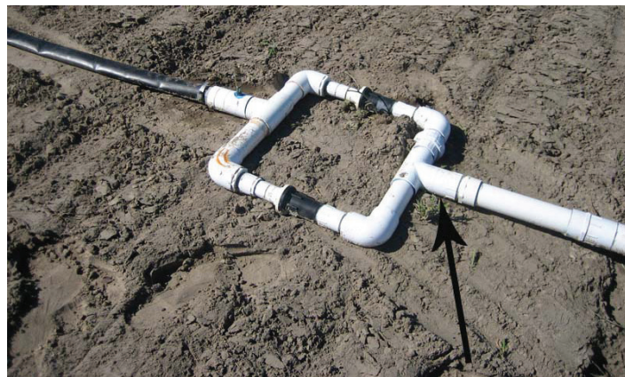
Figure 7. Pressure regulators are installed side-by-side in this system to allow a greater flow rate. Note the small injection port for chemical injection.
