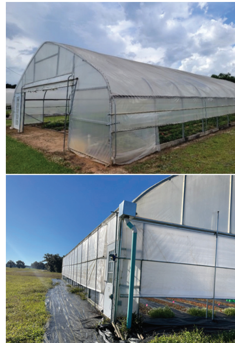
Figure 4. A single-bay high tunnel with roll-up sidewalls and end walls operated manually (top) vs. a multi-bay high tunnel with an automated control system for sidewall and end wall ventilation based on inside air temperatures (bottom).
