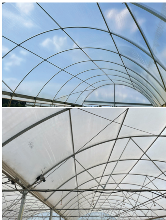
Figure 5. High tunnels covered with a single layer (top) vs. double layers (bottom) of polyethylene film. Credits: Shufang Tian, UF/IFAS
