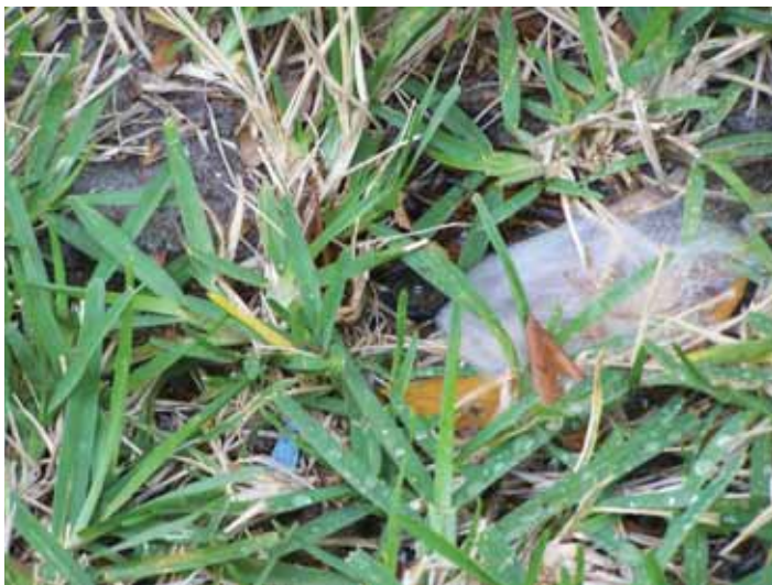
Figure 7. Spray head that no longer pops-up causing irrigation to only reach turfgrass within a couple of inches of the spray. Credits: Michael Gutierrez
