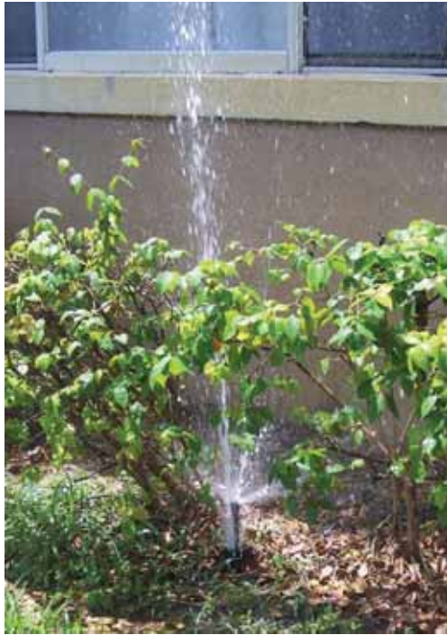
Figure 4. Leak in a spray due to a worn seal. Credits: Ernesto Clark
