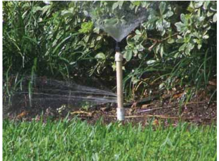
Figure 15. Pipe leak located below a spray head. Credits: Michael Gutierrez
