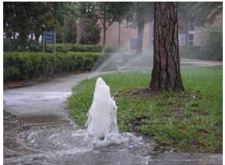
Figure 11. Nozzle on the sprinkler has been knocked off or broken.
