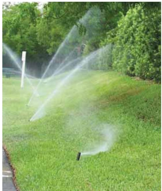
Figure 9. Tilted rotor spraying directly into turfgrass. Credits: Michael Gutierrez
