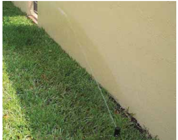
Figure 8. Rotor spraying water on the side of a house instead of the landscape.
