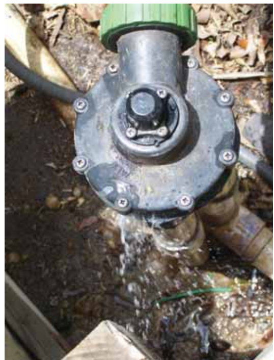
Figure 6. Leak in an indexing valve during irrigation due to high pressure in the system. Credits: Michael Gutierrez
