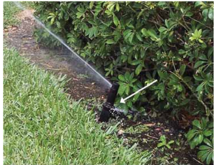
Figure 3. Leak in a rotor due to a worn seal indicated by the arrow. Note that the rotor body is crooked and should be buried to maintain vertical alignment and prevent damage from mowing. Credits: Ernesto Clark
