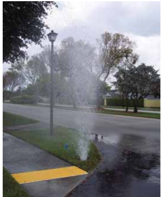
Figure 14. Large dramatic pipe leak. Credits: Ernesto Clark
