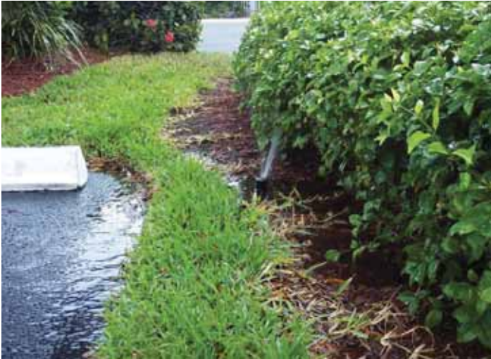
Figure 12. Irrigation system was designed before plants were installed. Modify system to meet plant needs. For established shrubs this sprinkler may not even be necessary. Credits: Mary McCready
