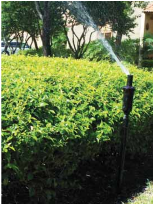
Figure 13. Riser added below rotor to give additional height so irrigation covers entire area. Credits: Michael Gutierrez
