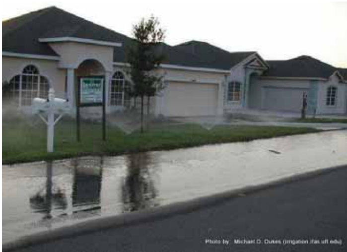
Figure 10. Wet area on pavement around landscaping due to poorly designed irrigation.
