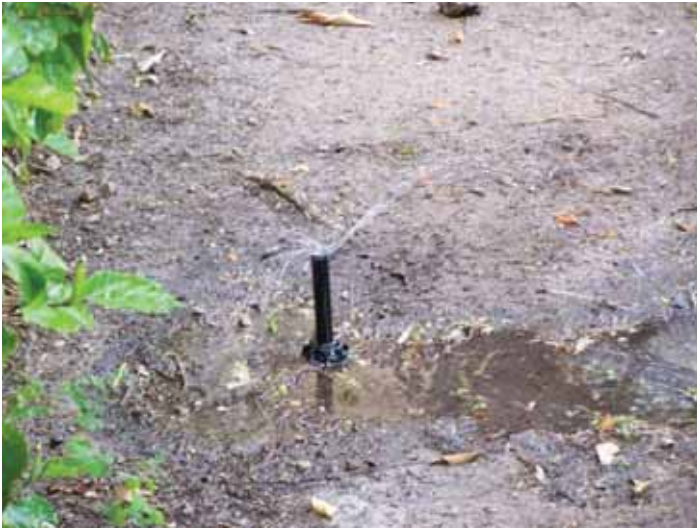
Figure 1. Picture of a clogged spray type sprinkler. Credits: Michael Gutierrez
