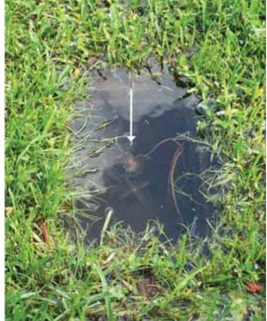
Figure 5. Leaking solenoid valve (indicated by arrow) covered in water after irrigation. Credits: Michael Gutierrez
