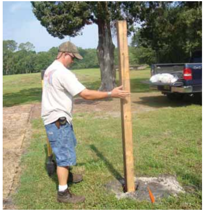
Figure 5. Hole for the supporting structure. Credit: B. M. Santos and T. P. Salame-Donoso, UF/IFAS
