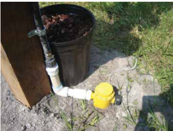
Figure 9. Install water timer (optional). Credit: B. M. Santos and T. P. Salame-Donoso, UF/IFAS
