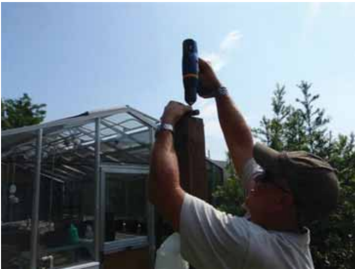
Figure 7. Install irrigation pipes on top of each pole. Credit: B. M. Santos and T. P. Salame-Donoso, UF/IFAS
