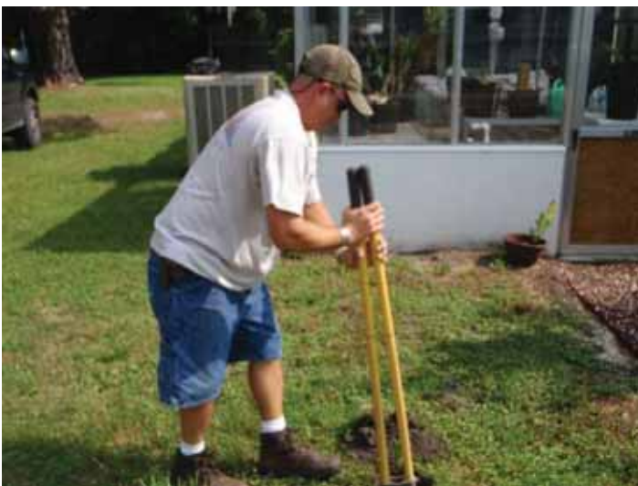
Figure 4. Dig a 2 ft hole. Credit: B. M. Santos and T. P. Salame-Donoso, UF/IFAS
