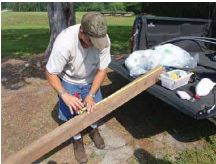
Figure 3. Measure the underground 2 ft of the pole. Credit: B. M. Santos and T. P. Salame-Donoso, UF/IFAS
